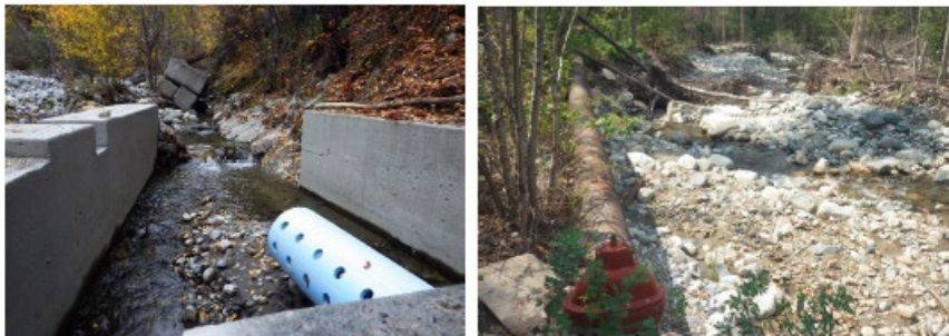
Figure 2 Shuttleworth POD infrastructure photos looking upstream (left) and downstream (right)
