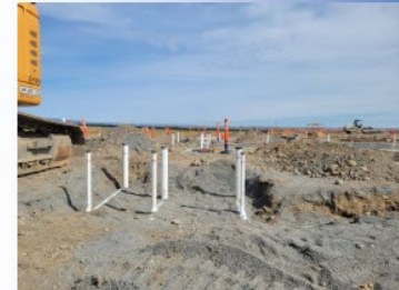
Building A Underground Utilities
