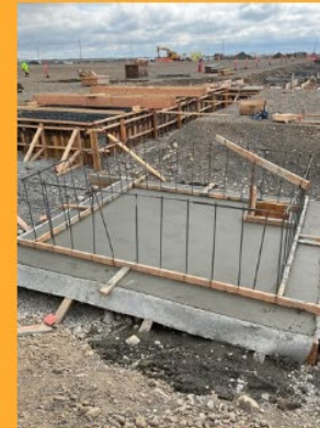
Building A Footings and Foundations
