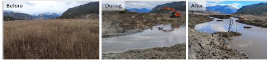
Fig. 2 Off-channel rearing habitat for Chinook, before, during, and after construction.
