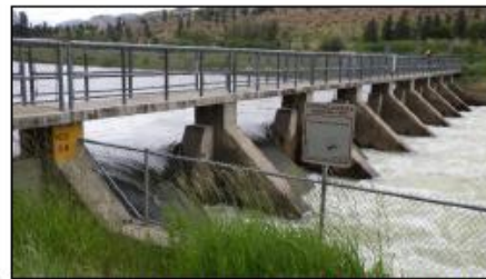
Example of existing VDS at high flow (80 m 3 /s).
