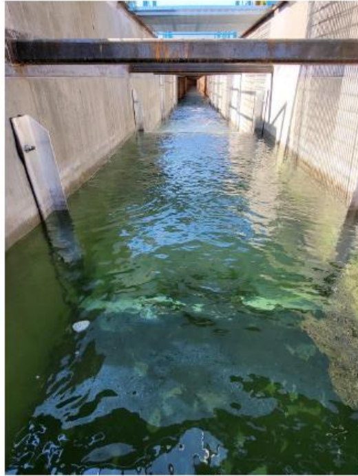
Looking downstream through fishway at stop logs
