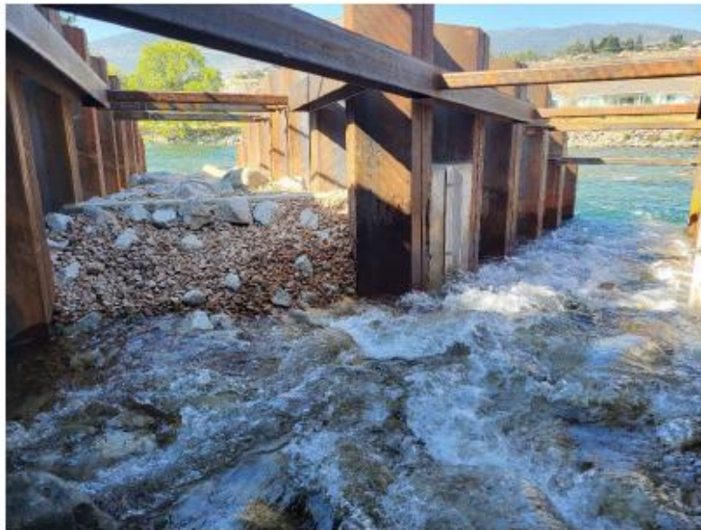
Looking downstream at both fish entrances (low and high flow)
