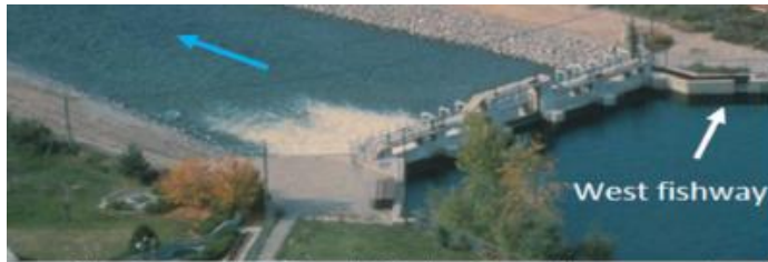
Photo: Okanagan Lake Outlet Dam. In 2019, the existing west fishway was opened allowing migrating fish to enter Okanagan Lake.
