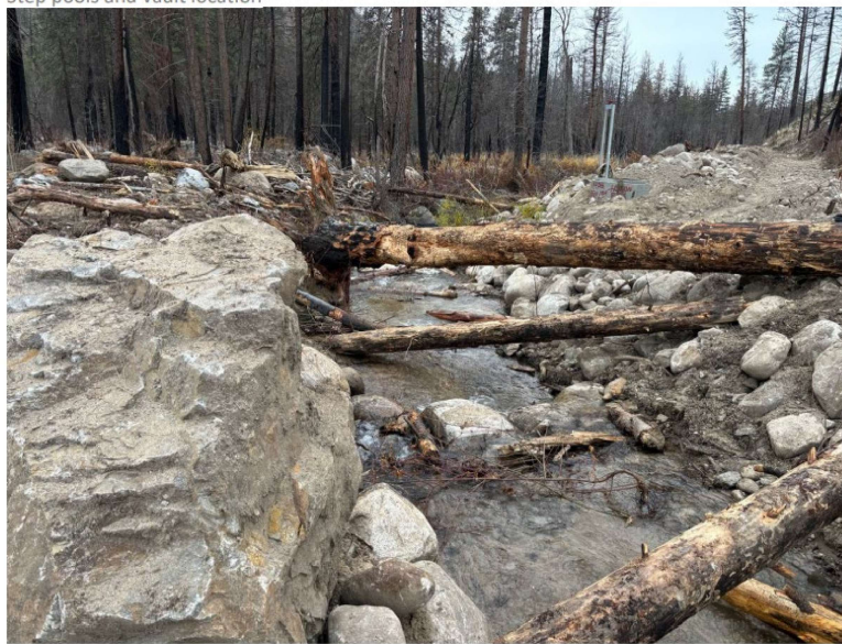
Step pools and vault location
