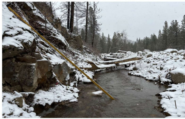
Macpherson side channel supply, irrigation pipe buried and ballasted under creek.
