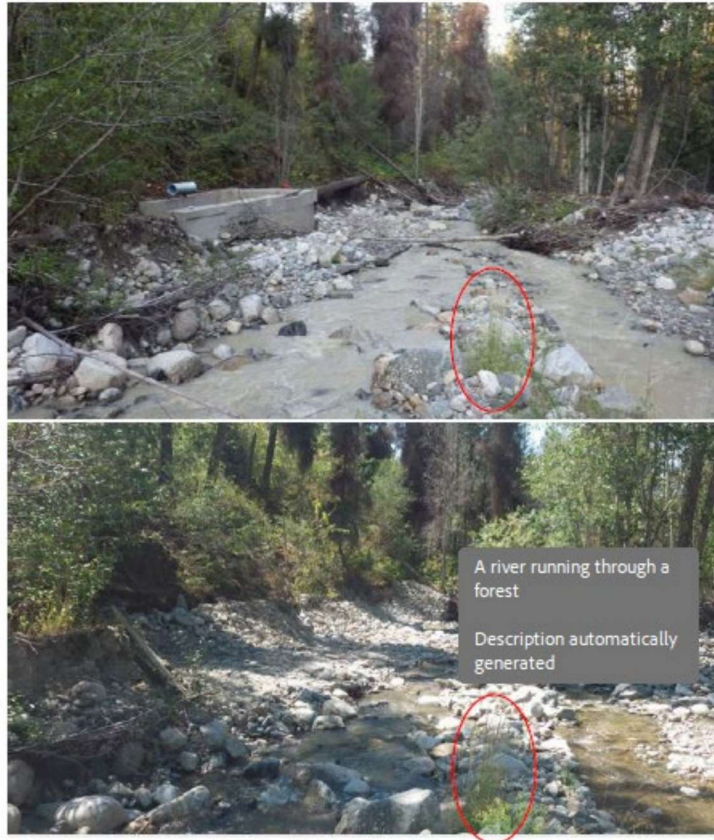
Figure 3 Top: Preconstruction photo of diversion infrastructure August 6 th , 2024. Bottom: Postconstruction photo of diversion infrastructure site looking downstream at re graded left bank August 7 th , 2024. An undisturbed patch of grass is highlighted as a reference point in both photos.
