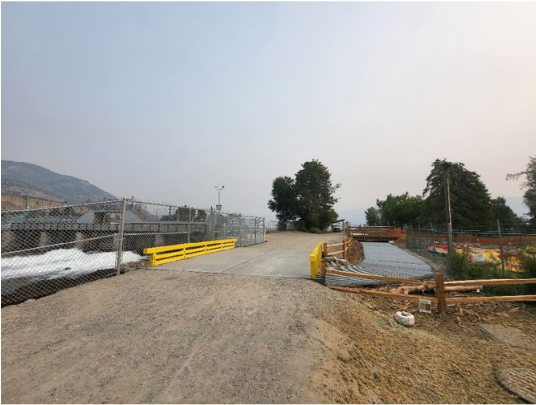
Looking north towards Okanagan Lake at vehicle and pedestrian bridges.
