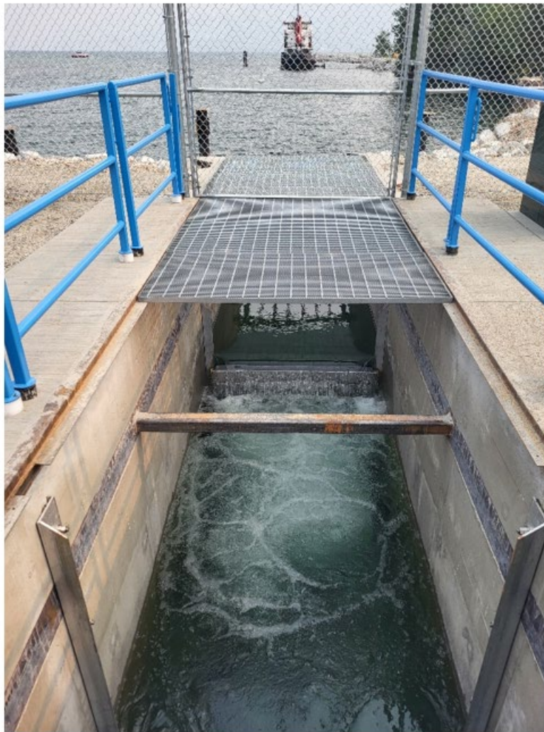
Looking down at top stop log, north end into Okanagan Lake.
