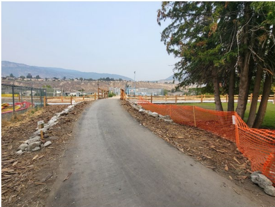
Pedestrian bridge and approach. Hydroseeded and planting zones.
