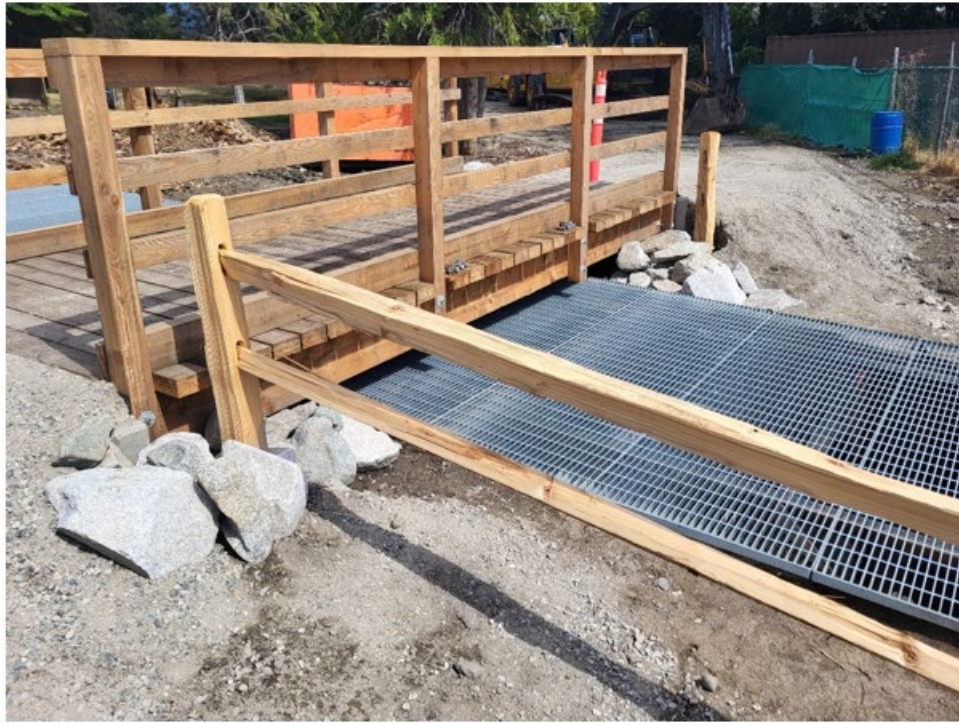
Pedestrian bridge, grating and fencing
