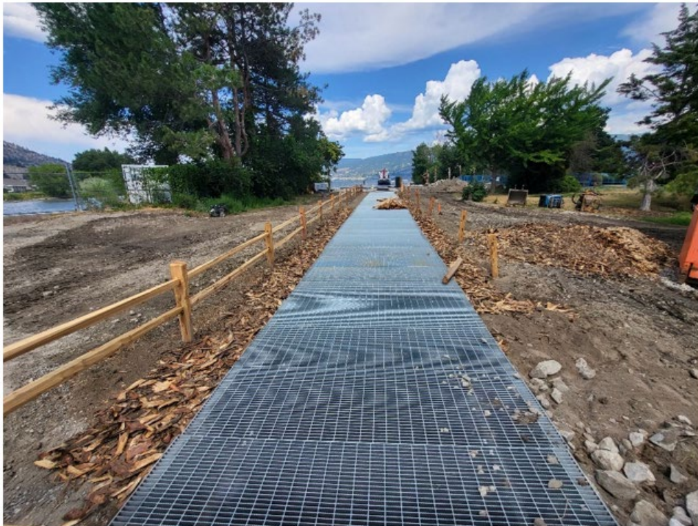
Grating, fencing (in progress) and mulch (in progress)
