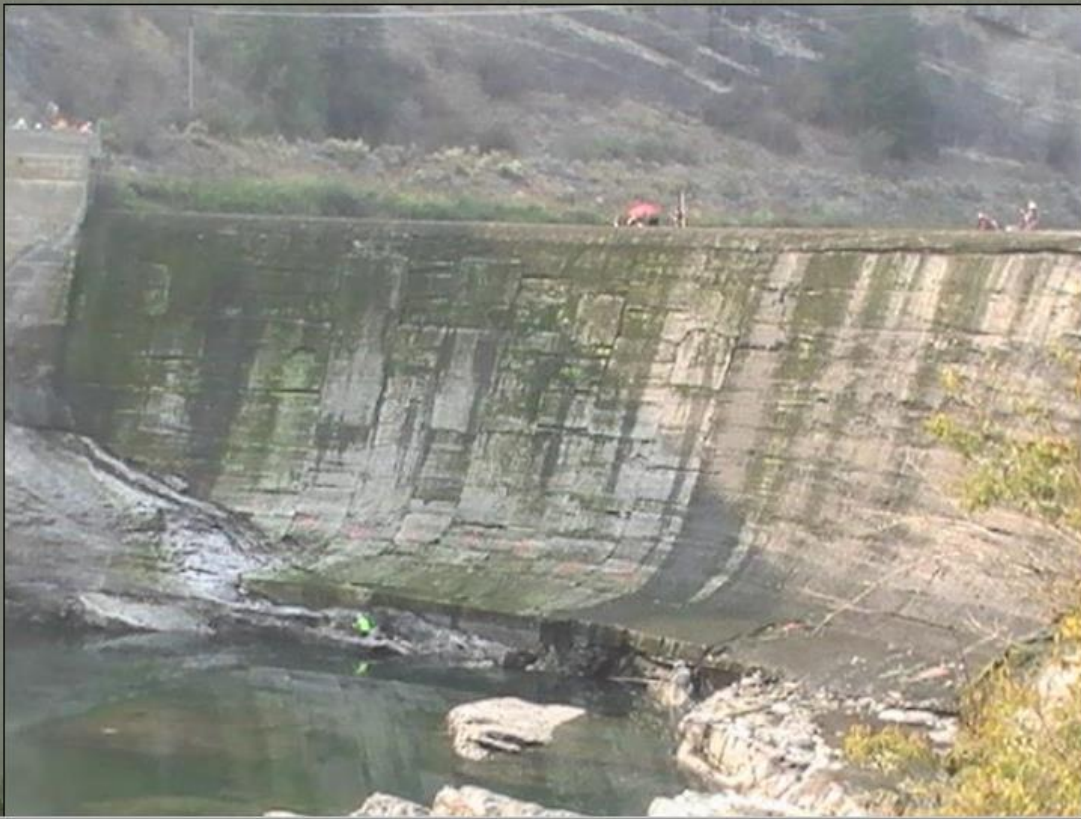
Image of Enloe Dam – dewatered – September 13, 2022
