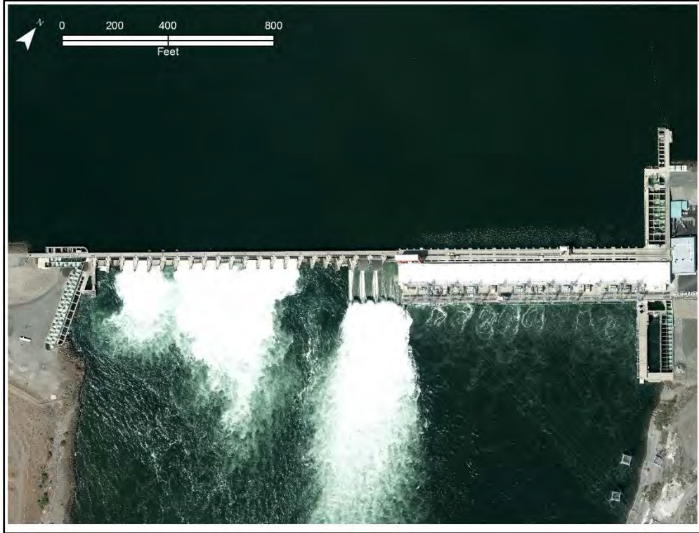
Figure 2 Aerial photograph of Priest Rapids Dam, Priest Rapids Hydroelectric Project, mid-Columbia River, WA.
