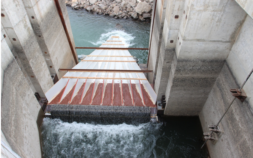
Figure 3 Wanapum Left Bank Fishway Exit Passage System. Completed and operational on April 15, 2014.
