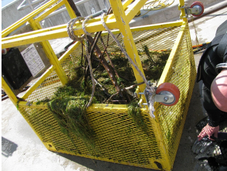
Figure 6 Photograph of typical aquatic vegetation and debris that is removed from the pump intake screens or the auxiliary water supply system.
