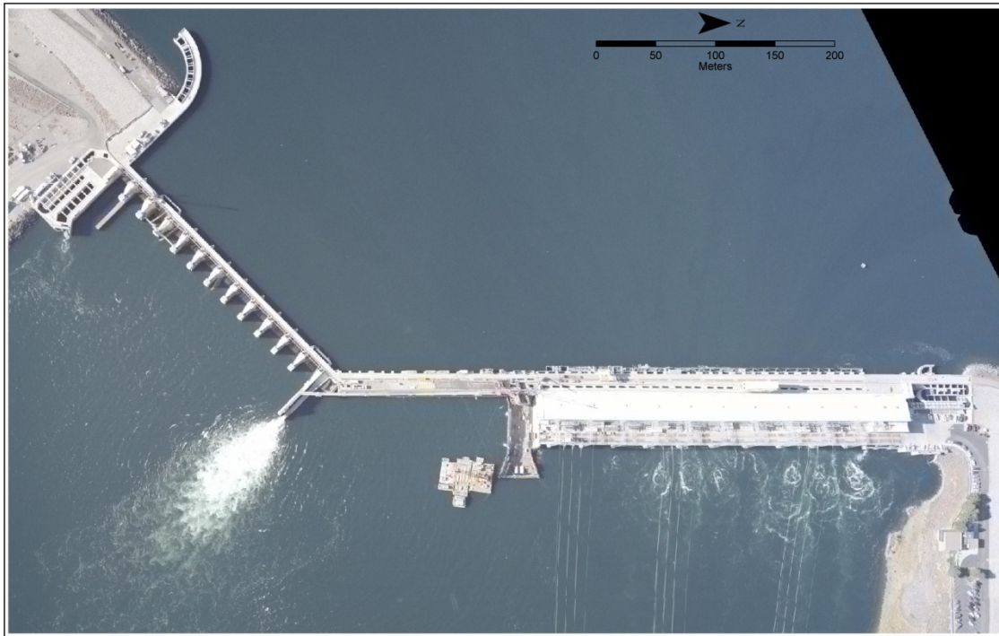
Figure 5 Aerial photograph of Wanapum Dam, mid-Columbia River, WA.
