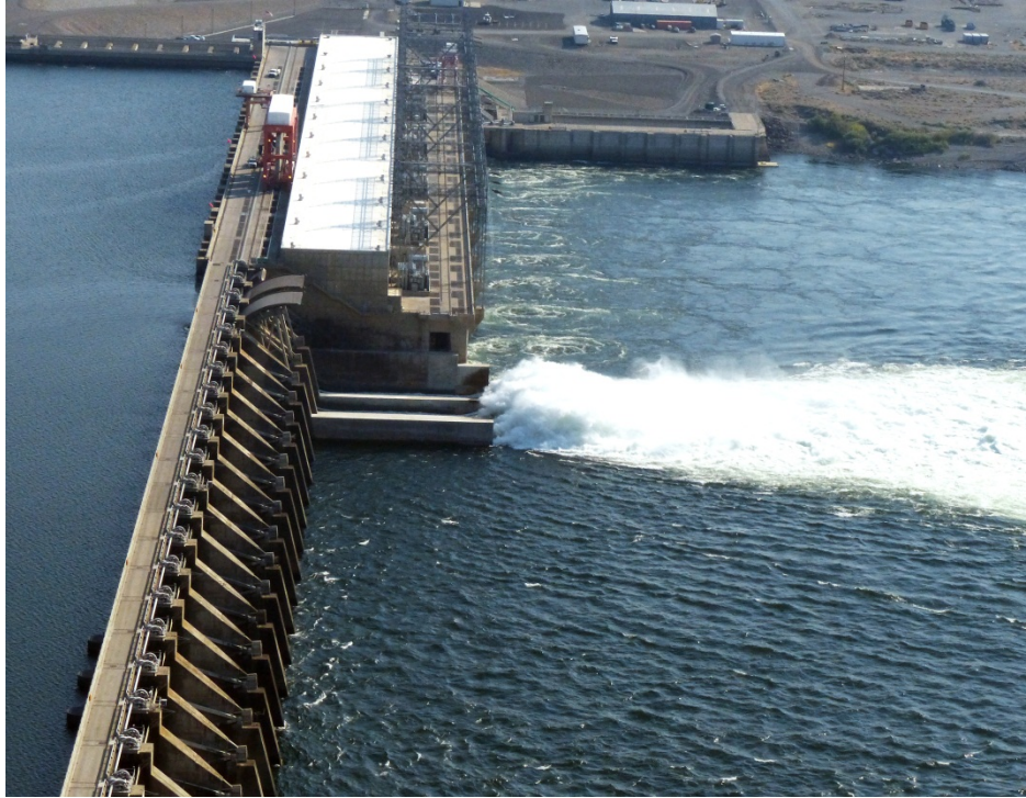
Figure 8 Priest Rapids Fish Bypass in operation, April 2014.
