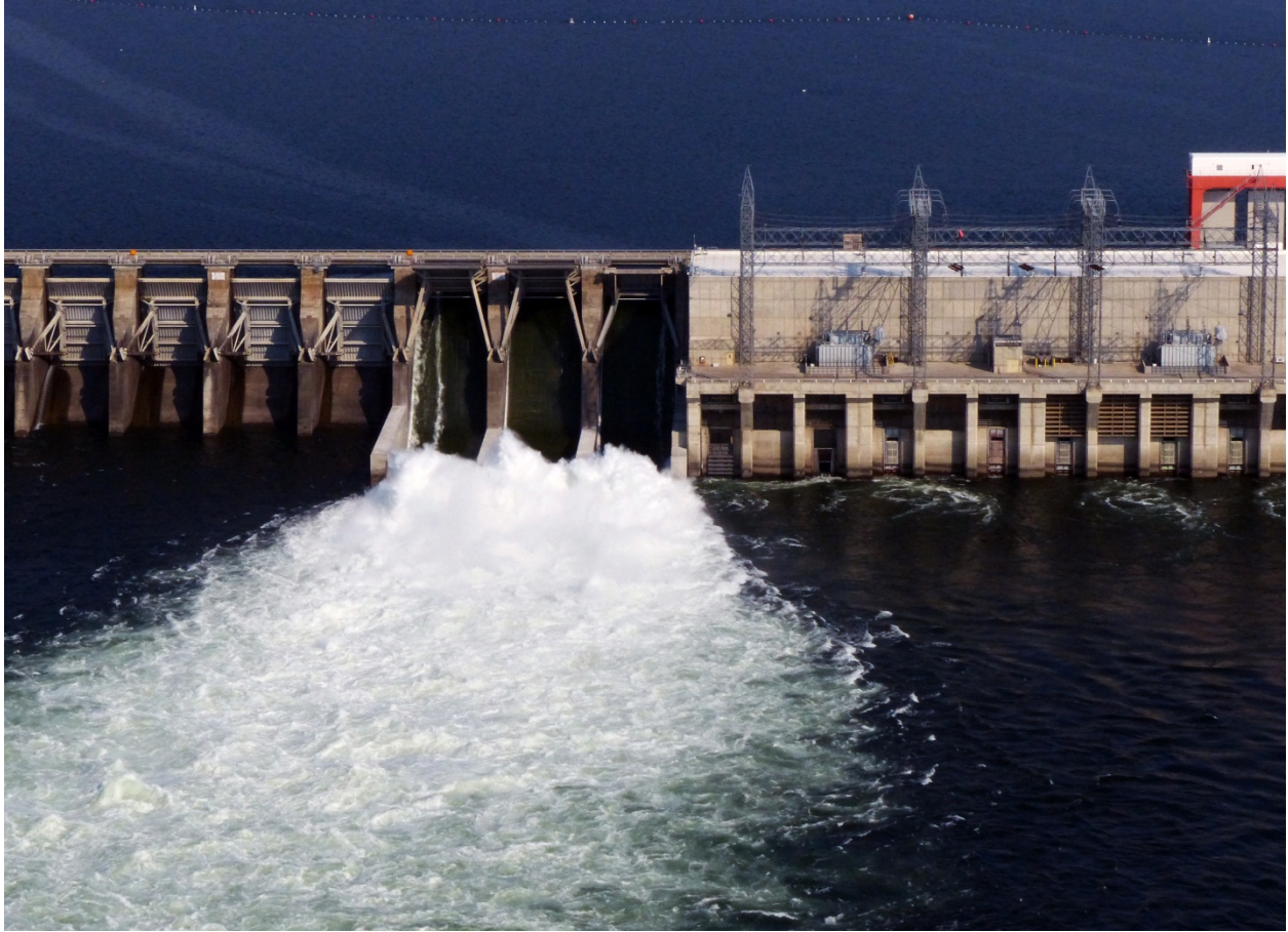
Figure 7 Priest Rapids Fish Bypass in operation, looking upstream at gate(s) and spillway improvements, April 2014.
