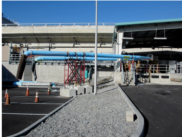
Figure 12 Additional modification implemented at the Priest Rapids Off-Ladder Adult Fish Trap on May 22, 2014 to allow for multi-truck loading.
