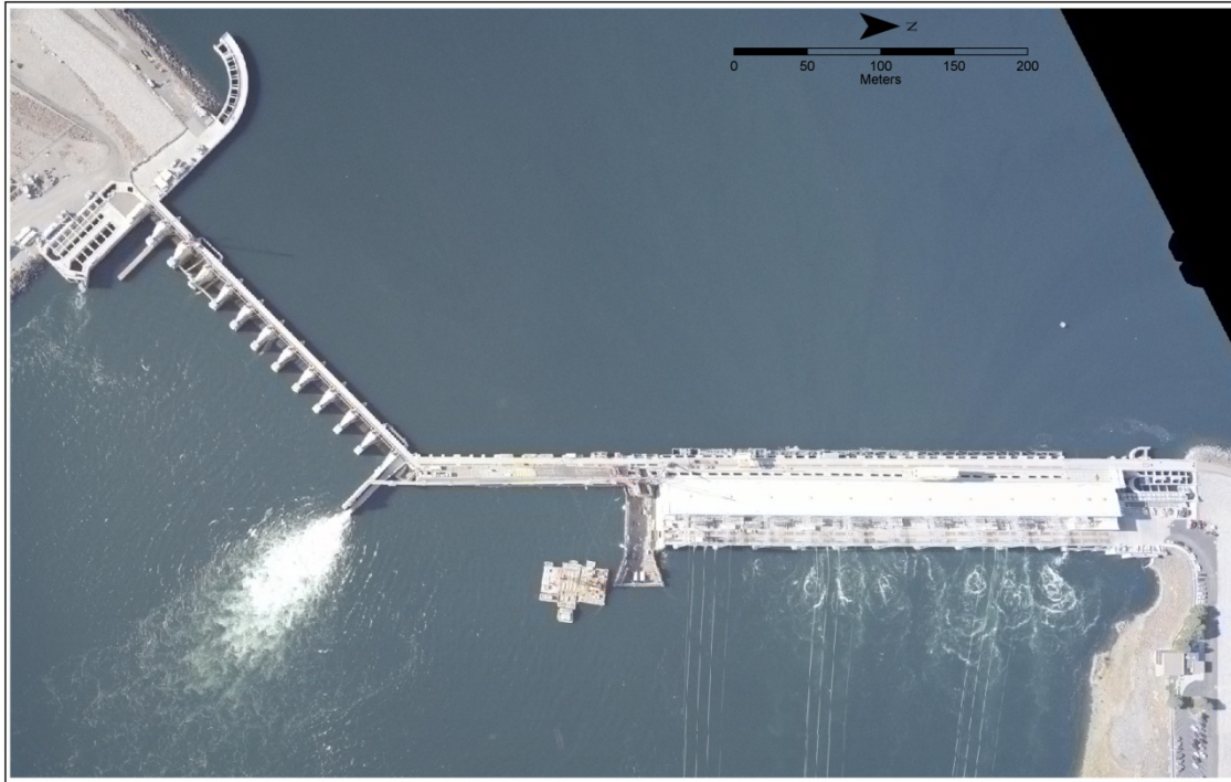
Figure 2 Aerial photograph of Wanapum Dam, mid-Columbia River, WA
