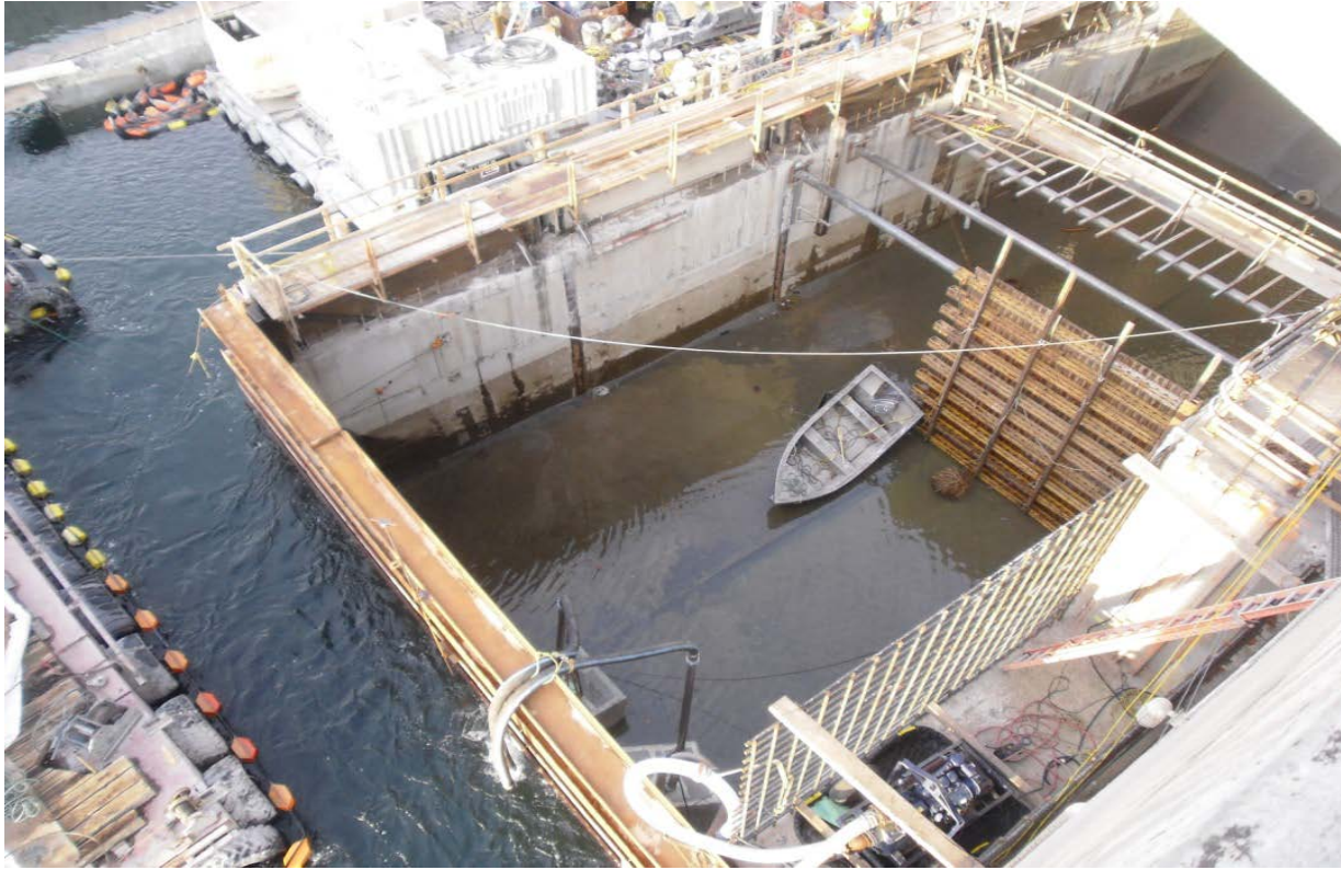
Figure 5 Priest Rapids Fish Bypass – Spill bay 22 dewatering.
