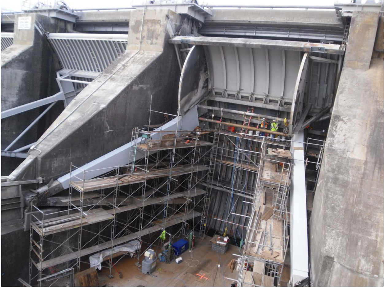
Figure 4 Priest Rapids Fish Bypass – Gate 22 Modifications, 2011.
