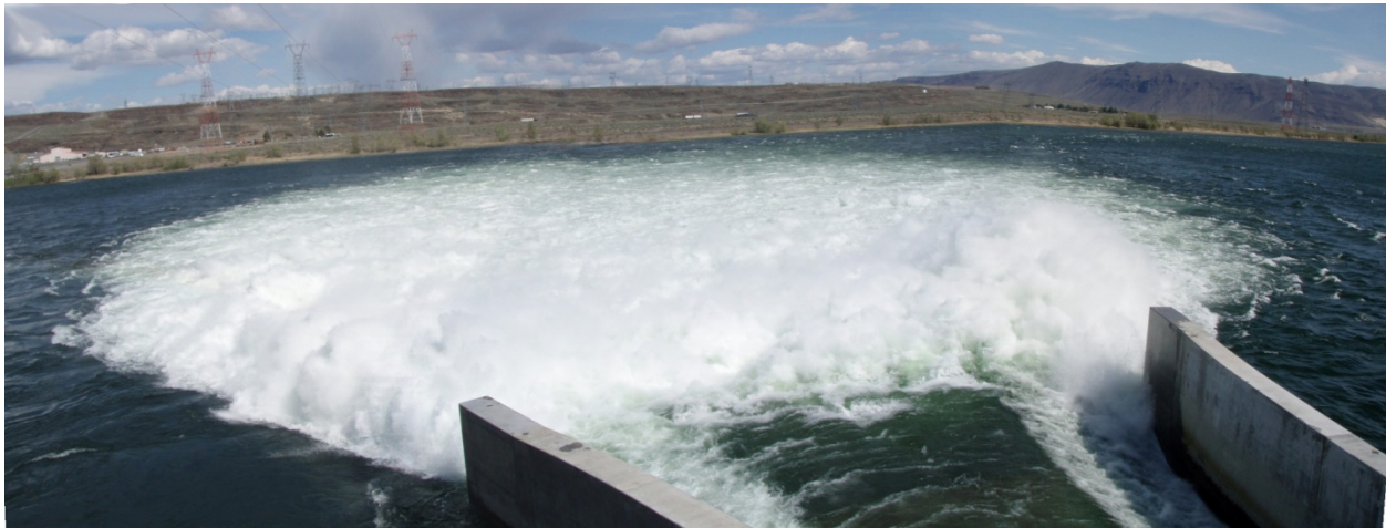
Figure 3 Photograph of Wanapum Fish Bypass facility, looking downstream, mid-Columbia River, WA
