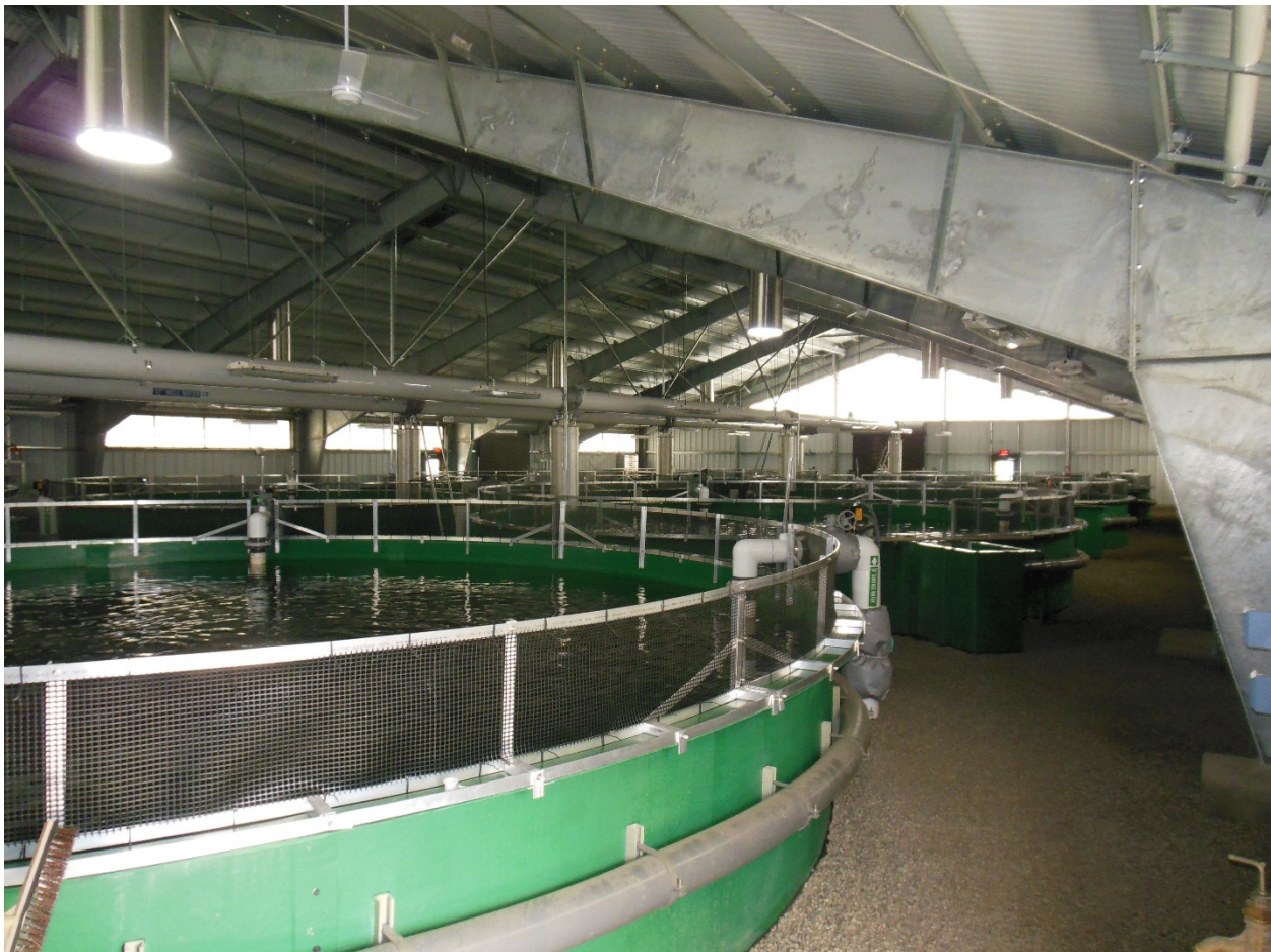
Figure 9 Carlton Acclimation Facility rears Methow summer Chinook using eight 30-foot diameter round tanks.
