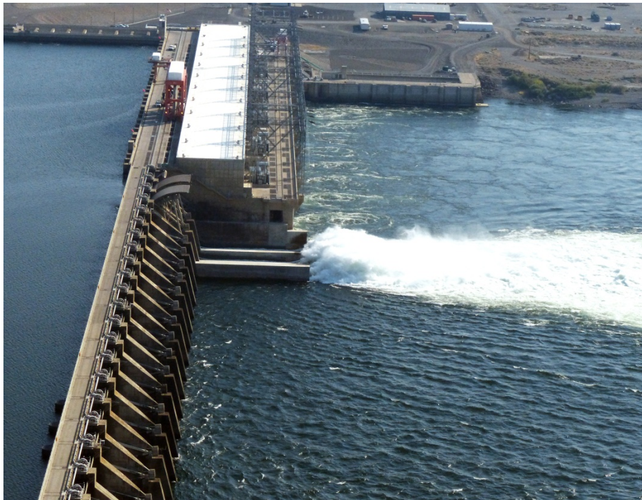
Figure 3 Priest Rapids Fish Bypass in operation, April 2014.
