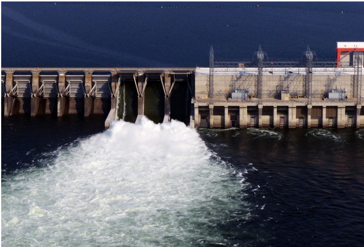
Figure 4 Priest Rapids Fish Bypass in operation looking upstream at gate(s) and spillway improvements, April 2014.
