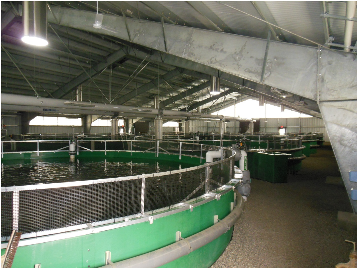
Figure 11 Carlton Acclimation Facility rears Methow summer Chinook using eight 30 foot round tanks.
