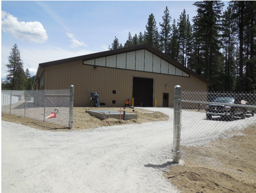
Figure 9 Nason Creek Acclimation Facility.
