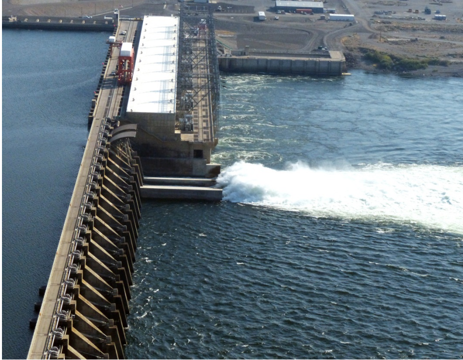
Figure 5 Priest Rapids Fish Bypass in operation, April 2014.
