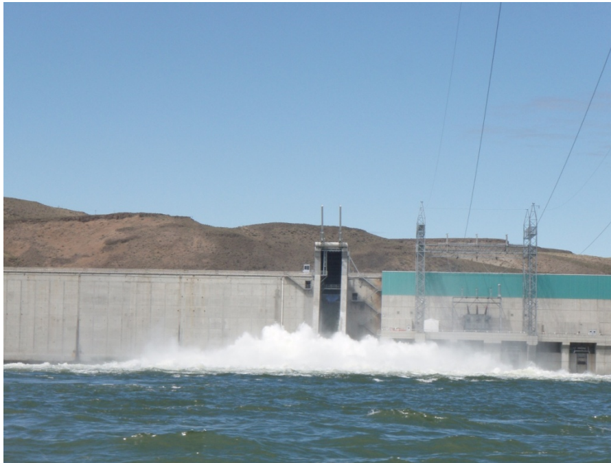
Figure 5 Photograph of the Wanapum Fish Bypass facility, mid-Columbia River, WA.
