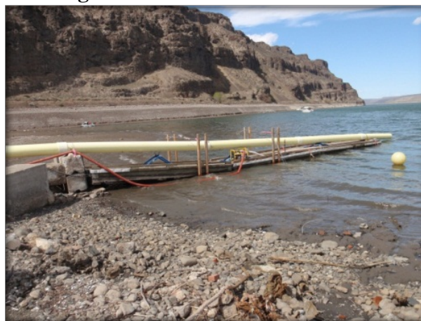
Figure 15 Rocky Coulee fish release pipe located upstream of Vantage, Washington.
