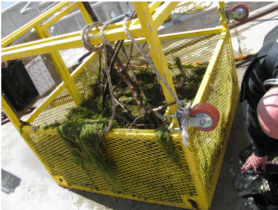
Figure 11 Photograph of typical aquatic vegetation and debris that is removed from the pump intake screens or the auxiliary water supply system.
