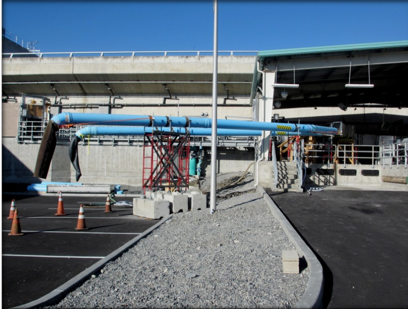
Figure 13 Additional modifications implemented at the Priest Rapids Off-Ladder Adult Fish Trap on May 22, 2014 to allow for multi-truck loading.
