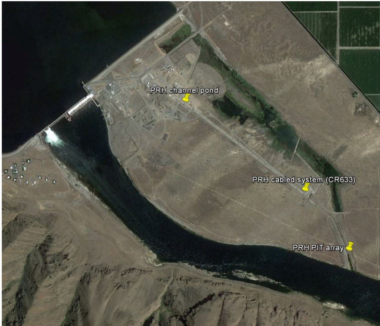
Figure 2.4. Google Earth image of Priest Rapids Dam that displays the channel pond in which acoustic-tagged fish were held following surgery and the cabled JSATS array (CR633) and PIT array that were located in the outflow channel to detect acoustic- and PIT-tagged fish as they migrated from the channel pond to the Columbia River.
