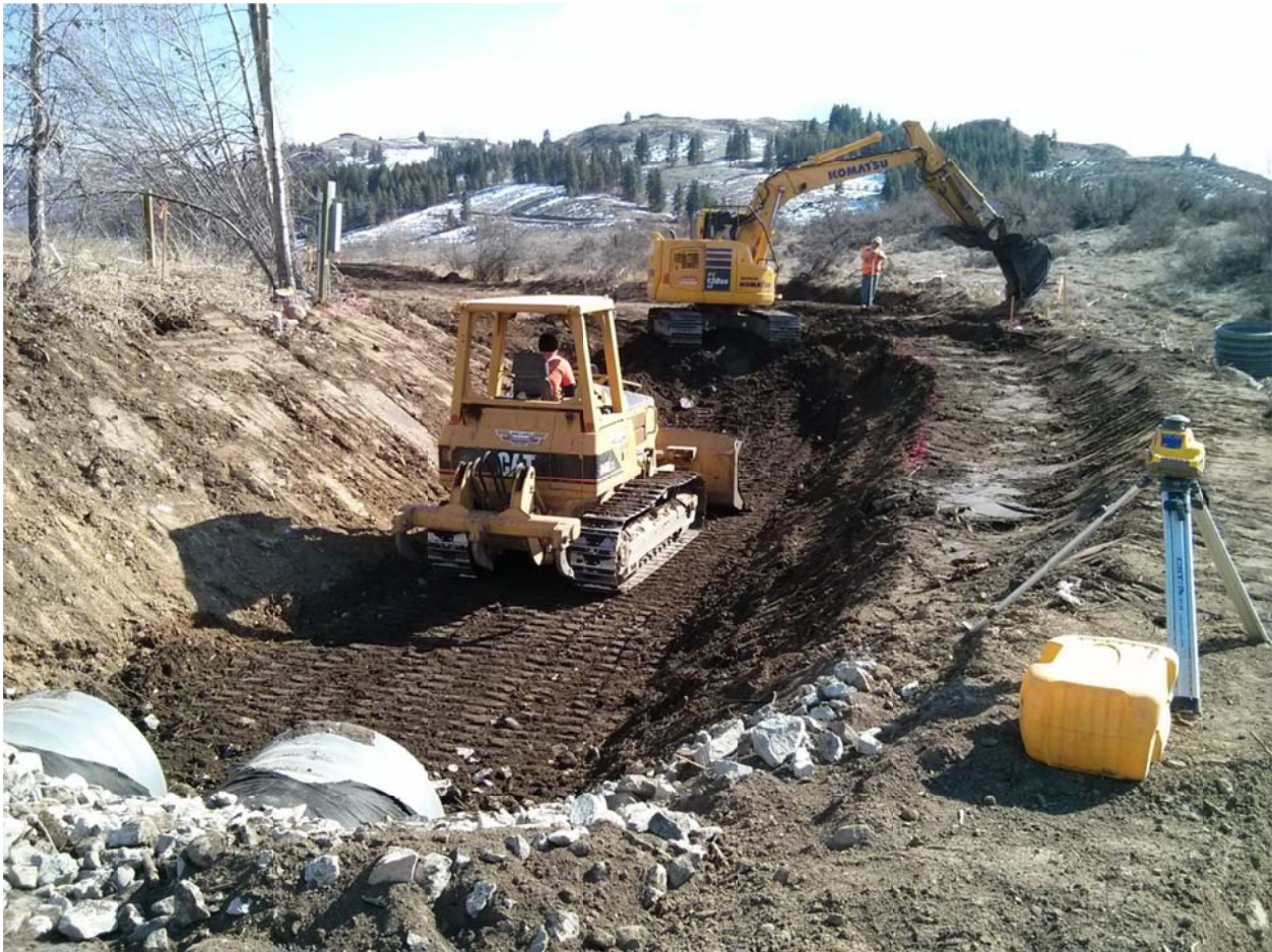
12. Reconstruction of the Chewuch Canal, below wright lateral pipe
