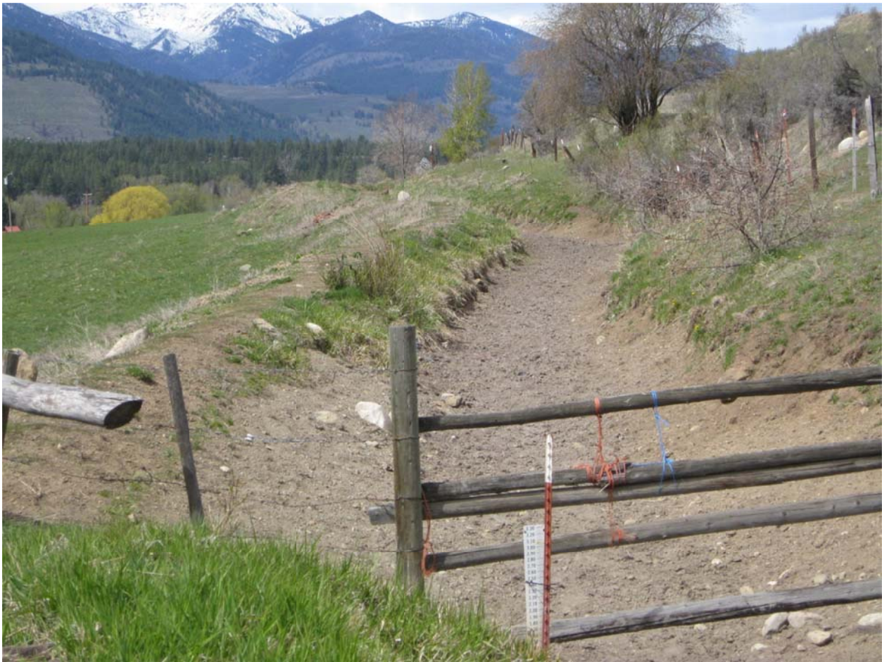
1. Chewuch Canal at Bear Creek, before project
