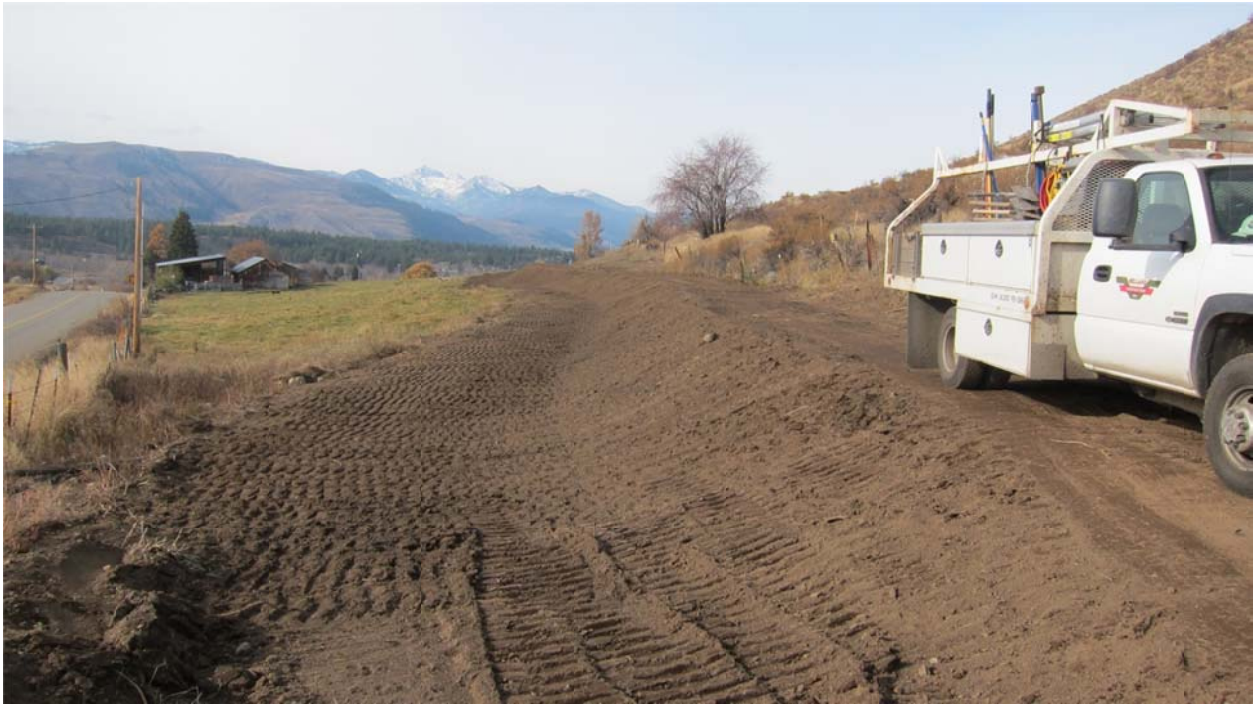
3. Chewuch Canal at Bear Creek after construction
