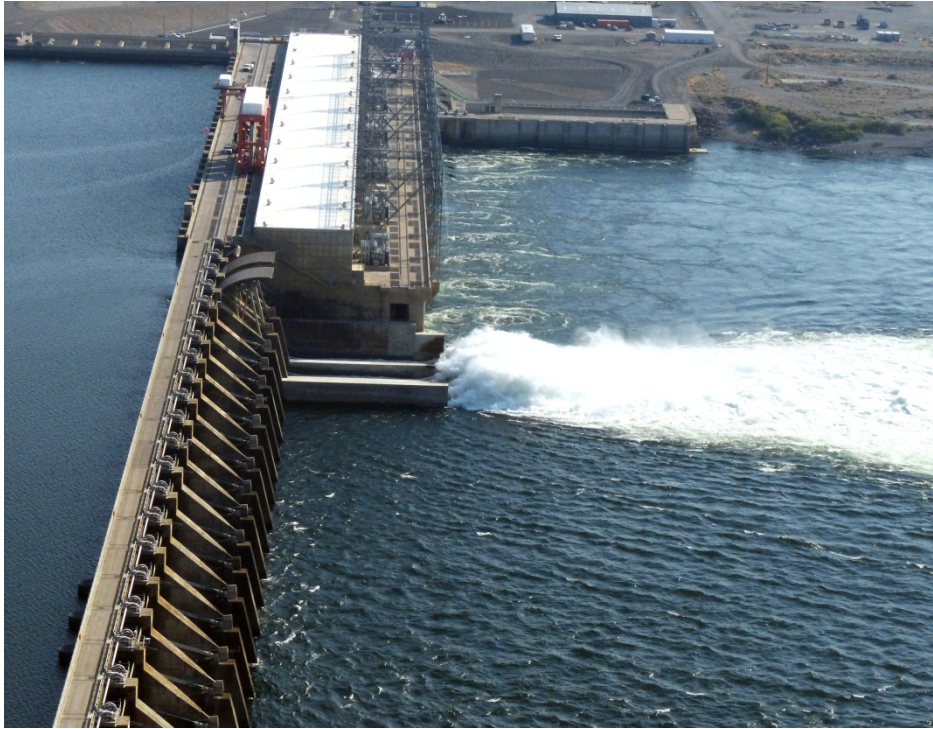
Figure 2 Priest Rapids Fish Bypass in operation, April 2014.
