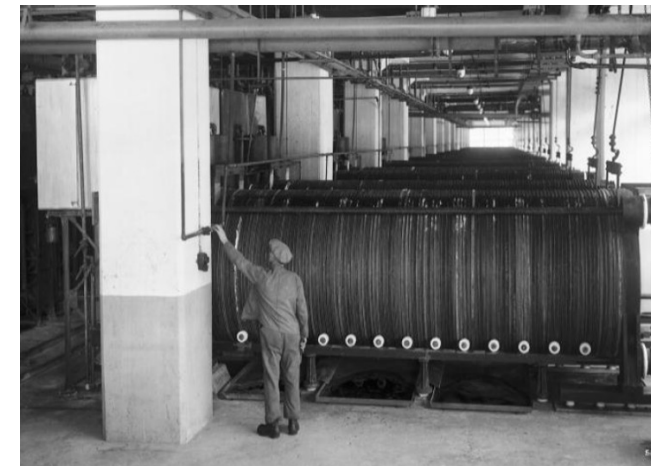
Rjukan Norway 32 MW electrolyzer, 1927-1970s
