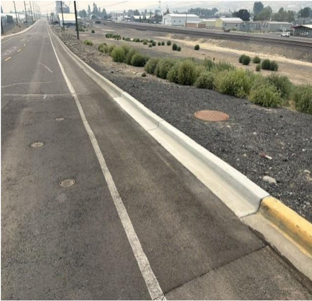
PRESSURE REDUCING VALVE ON A STREET NE
