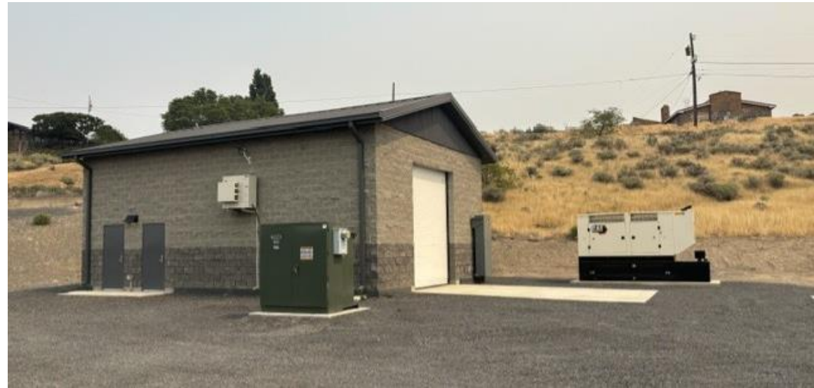
BOOSTER PUMP STATION
